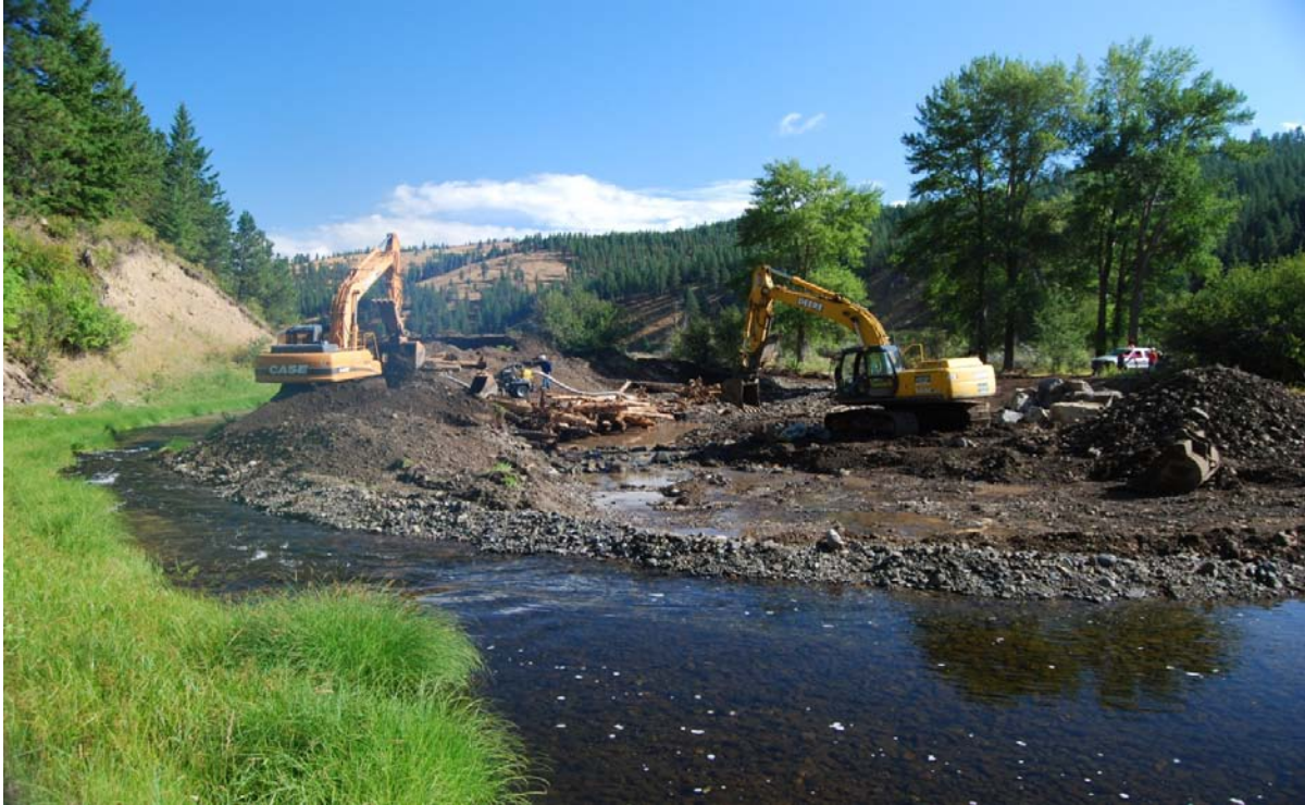
Figure 4. Heavy equipment preparing new channel.
