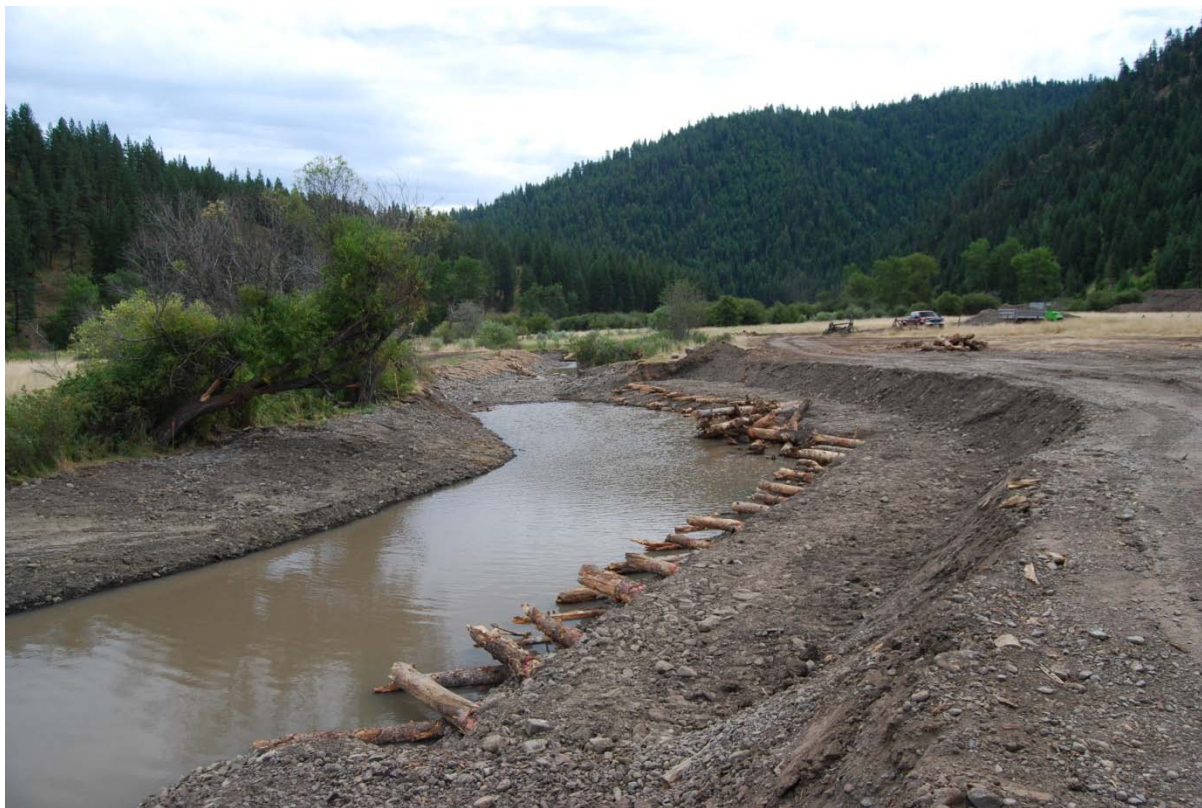
Figure 3. View of new channel and embedded log structures.
