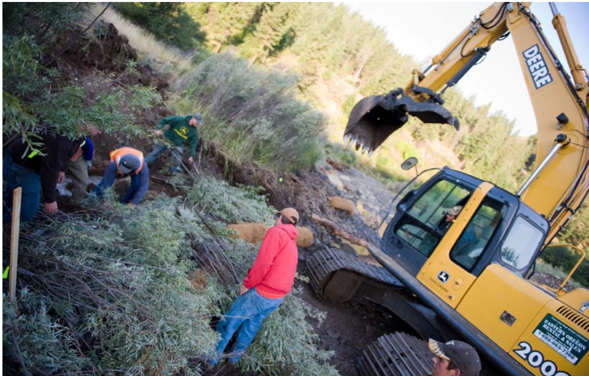
Figure 2. Preparation for channel realignment
