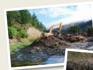
Above: Habitat construction underway on the Middle Fork. 3
