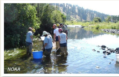
Crews catch and relocate fish to prevent them from being harmed by construction of a restoration project.
